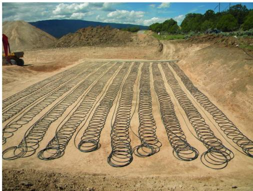
There are two categories of systems: horizontal and vertical loops. Horizontal loops (as in the image to left) involve pipe laid horizontally and require more space, but are less expensive to put in. This heat and cooling technology is often installed into new schools where the exchange pipe can be laid directly under playing fields during construction.
